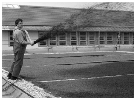
Hydroseeding an extensive green roof.
